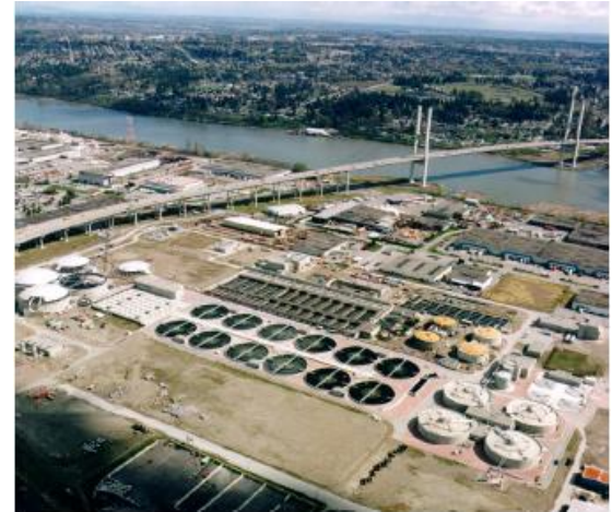
Annacis Island WWTP, Delta, BC, Canada
