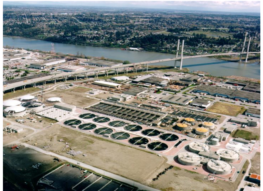
Annacis Island System Site
