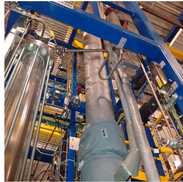
Oil Upgrading System
