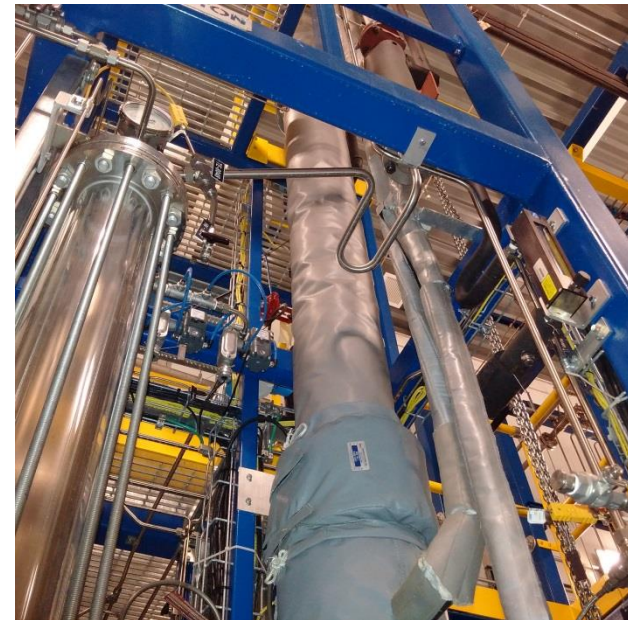
Oil Upgrading System
