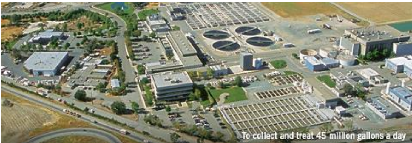
Central San System Site
