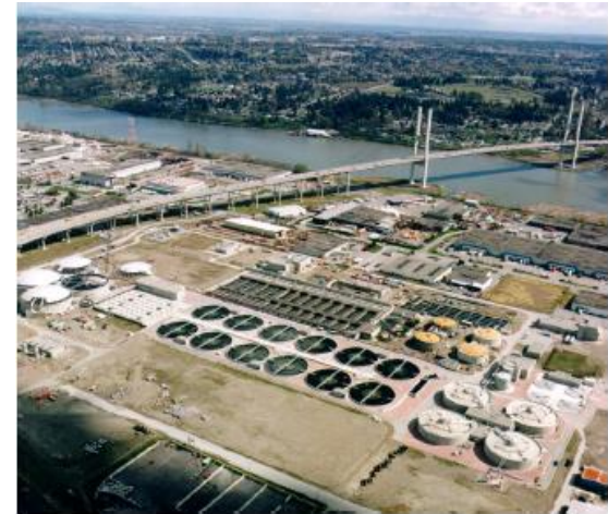
Annacis Island WWTP, Delta, BC, Canada
